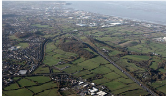
Avonmouth Severnside Enterprise Area flood defence project.
