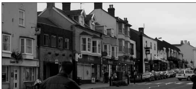
Shop front details are critical
