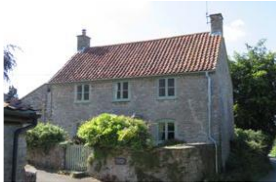
Detached two storey dwelling abutting the road on a perpendicular orientation. Stone walling with pantile roof. Low stone boundary wall to front garden.
