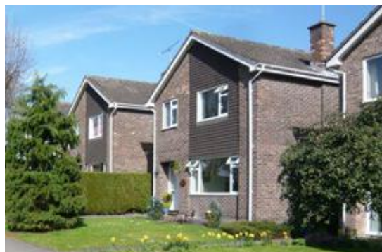
Detached dwelling from the 1970s, with brick and hanging tile facades.
