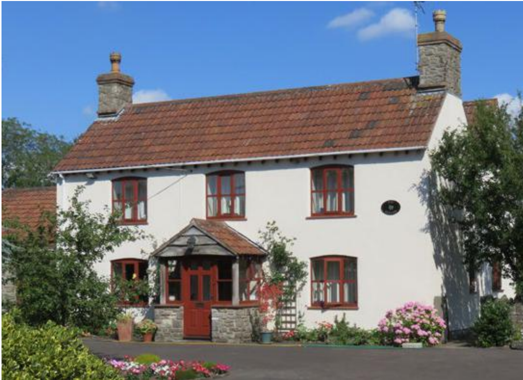
Rendered detached dwelling with stone and timber detailing to the porch. Wide fronted, narrow depth with low pitched roof. Further example of pantiles. Property abuts the street with minimal setback.
