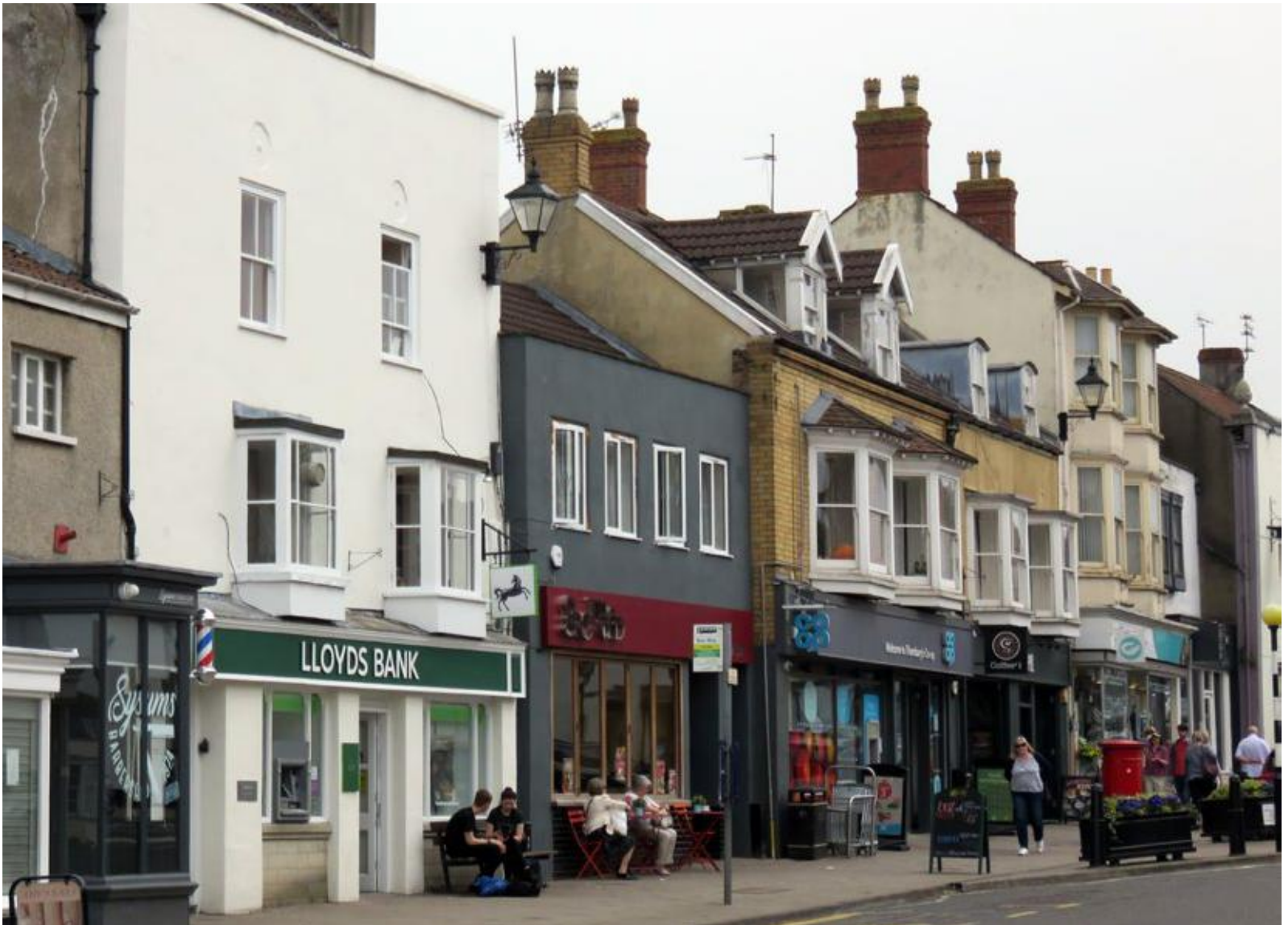
View of high street shows properties abutting the footway to create good levels of enclosure. Window bays and dormers form a lasting characteristic of the original properties, whilst shop front signage introduce a consistent horizontal emphasis along the frontage.
