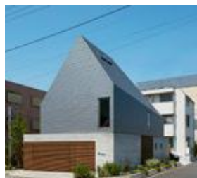
Tile and slate hanging
