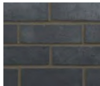
Blue brick plinths
