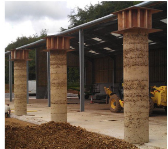
Rammed earth columns at Drawing Matter, Somerset.
