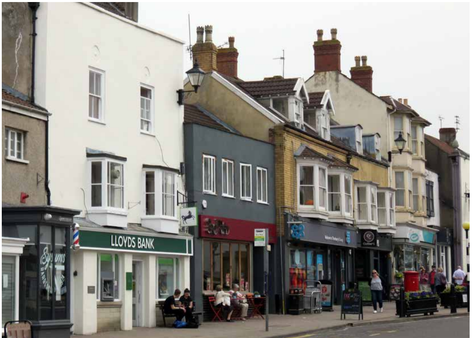
View of high street shows properties abutting the footway to create good levels of enclosure. Window bays and dormers form a lasting characteristic of the original properties, whilst shop front signage introduce a consistent horizontal emphasis along the frontage.
