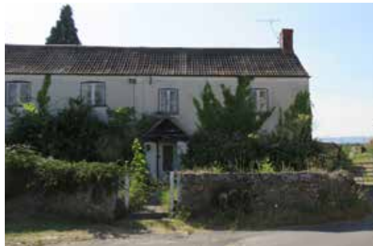
Wide fronted and narrow depth semi-detached dwellings with low roof pitch. Low stone wall to front garden.
