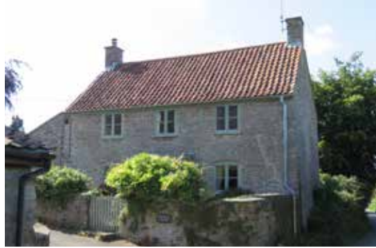
Detached two storey dwelling abutting the road on a perpendicular orientation. Stone walling with pantile roof. Low stone boundary wall to front garden.
