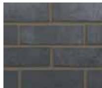
Blue brick plinths
