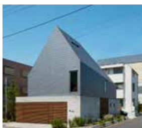
Tile and slate hanging
