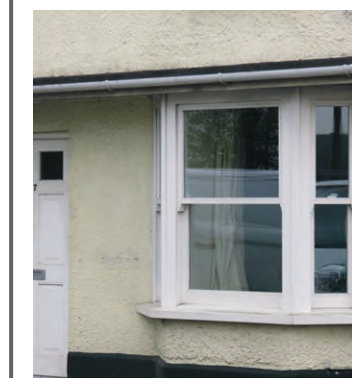
Ground level bays
