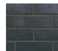
Blue brick plinths
