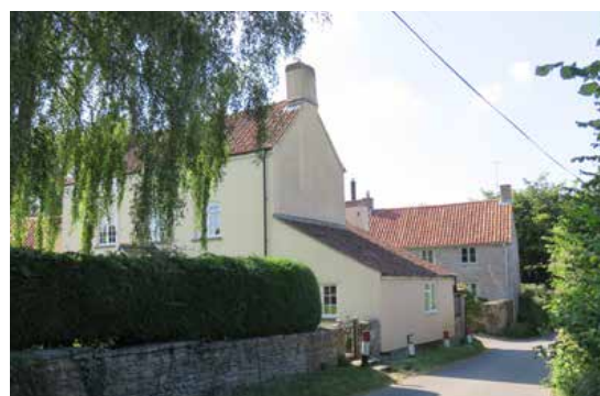
Further examples of properties siding onto the road, in this case with single storey lean-to creating variation and interest.
