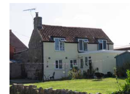
Examples of one and a half storey buildings with half-dormers on the first floor.
