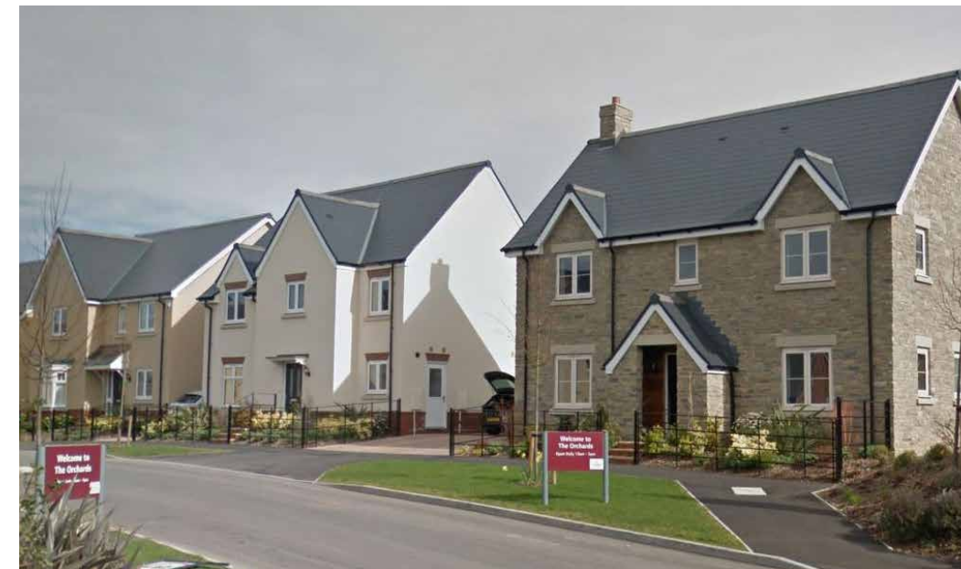
Post Farm: Detached family homes with varied use of stone and render walls with gabled features on the slate roofs.
