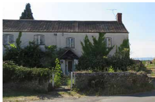
Wide fronted and narrow depth semi-detached dwellings with low roof pitch. Low stone wall to front garden.
