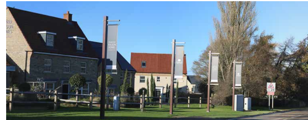
Park Farm: Development frontage set back from Butt Lane behind a planted grass verge helps to create an attractive gateway to the development and the town.
