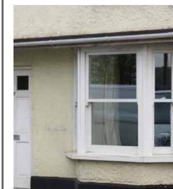
Ground level bays
