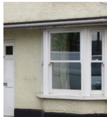
Ground level bays
