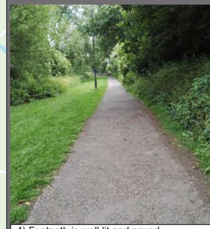
4) Footpath is well lit and paved, providing inclusive accessibility. Spot measurements taken on site show an average width of 2.0m.
