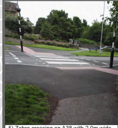
5) Zebra crossing on A38 with 2.0m wide footways on both sides of the carriageway.
