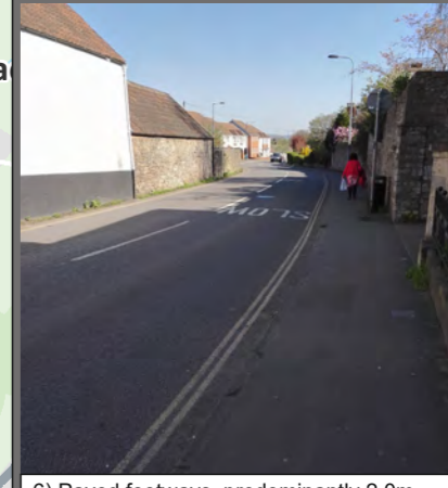
6) Paved footways, predominantly 2.0m in width, are provided from the pedestrian crossing to the high street on at least one side of the carriageway.
