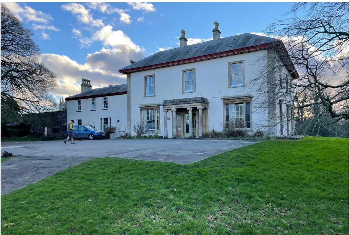
Image AC 22: View of the main north-east facing elevation of Sheiling School (from the north-east). It was built in the mid-1830s as Thornbury Park by Henry Wenman Newman.
