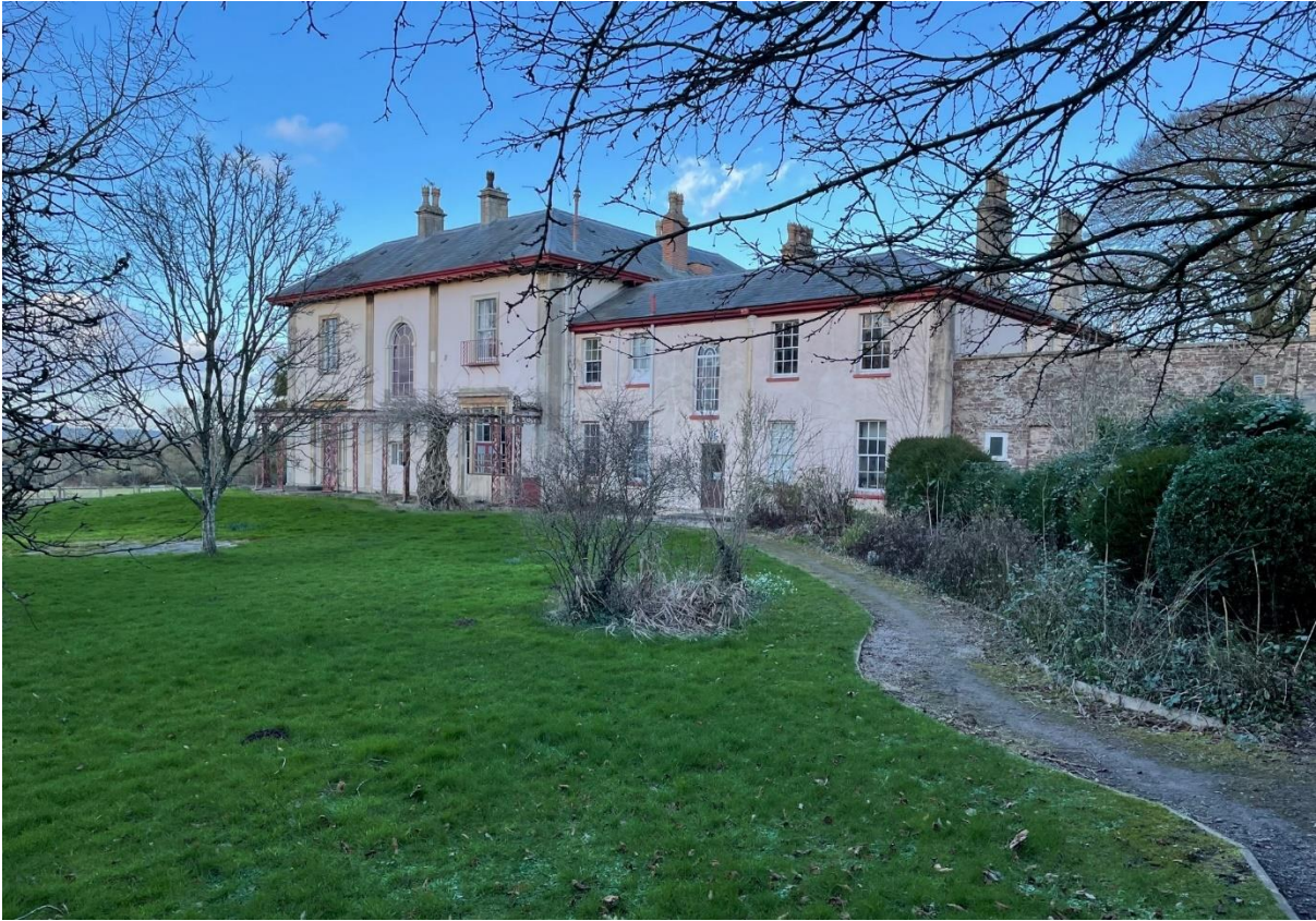
Image AC 23: View of the rear south-west facing elevation of Sheiling School (formerly Thornbury Park) looking north-eastwards.
