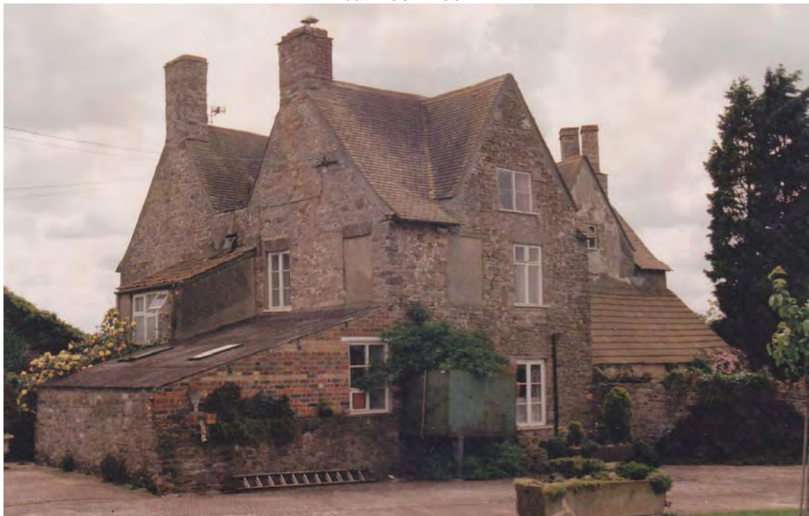
15 1994 north and east fronts with blocked kitchen windows and brick lean-to wall
