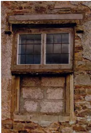
17 Detail of the stair tower with remains of blocked stone transom and c1900 timber leaded mullion; first floor 17th century timber ovolo mullion & blocked doorway in the rear lean-to (north wall)
