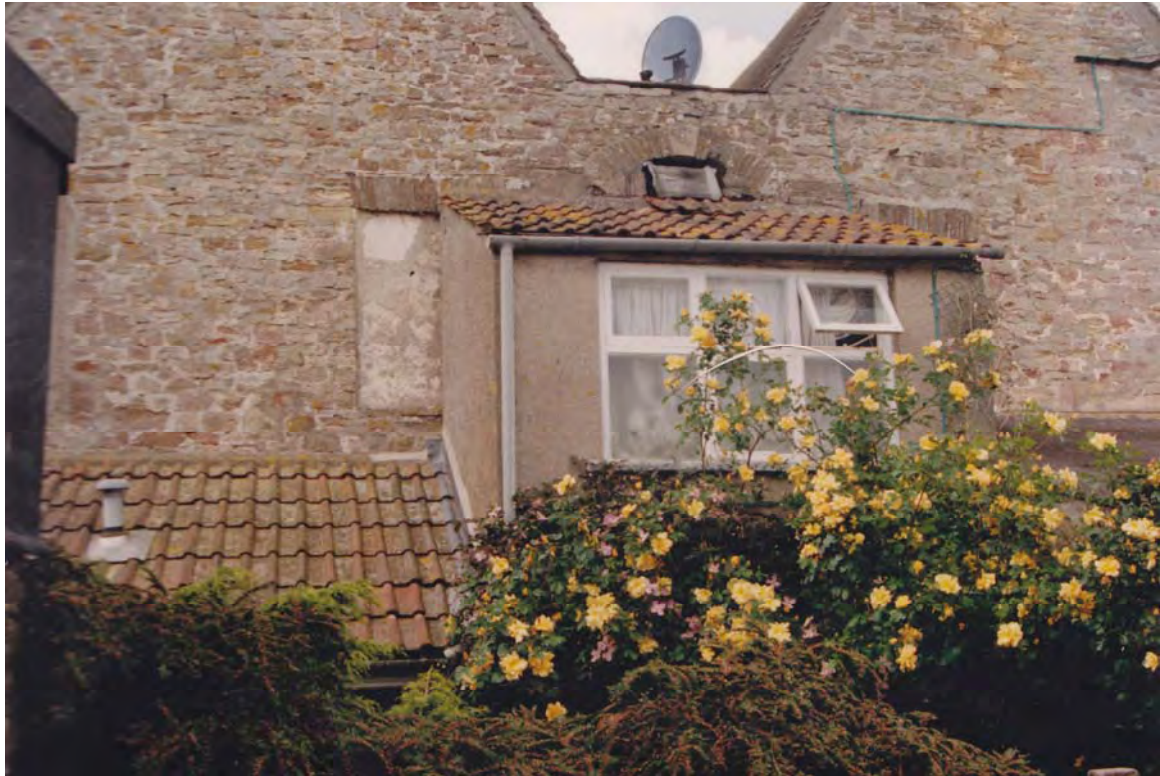
14 1994 Bathroom with larger casement & archway detail with valley gutter above bathroom roof
