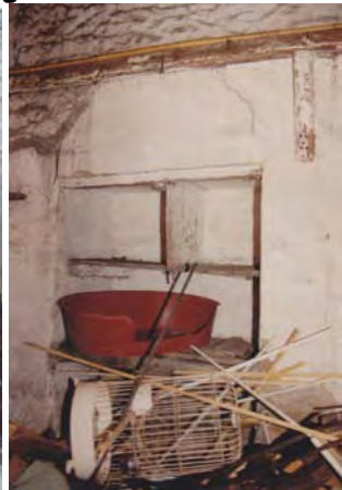
17 Detail of the stair tower with remains of blocked stone transom and c1900 timber leaded mullion; first floor 17th century timber ovolo mullion & blocked doorway in the rear lean-to (north wall)
