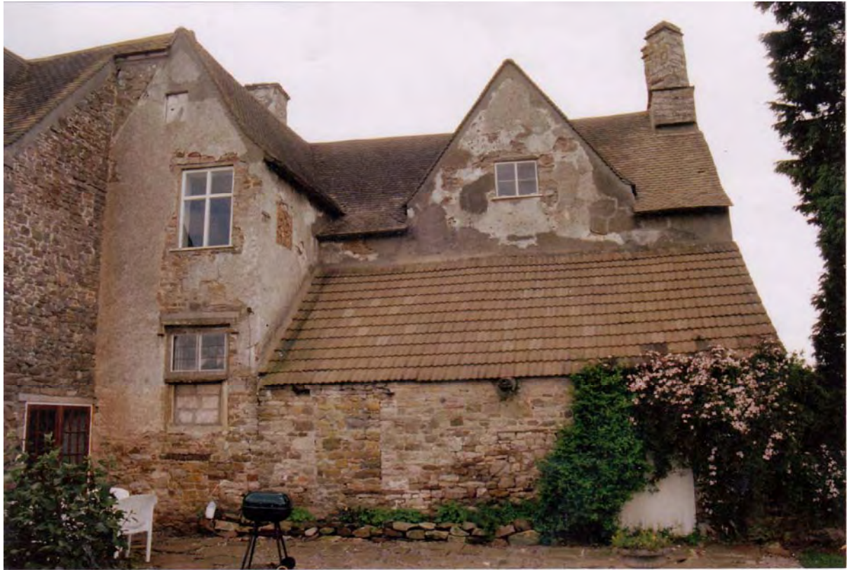
16 The North front showing the partially rendered gables with remains of a stone transom window in the stair tower and various blockages
