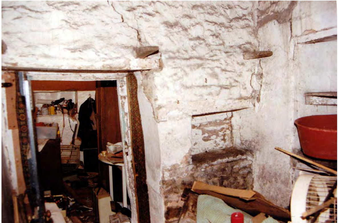
18 1994 Log Store with cheese rack brackets and keeping hole with blocked doorway and arch with further shelving
