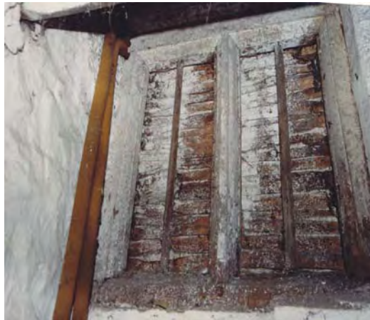
17 Detail of the stair tower with remains of blocked stone transom and c1900 timber leaded mullion; first floor 17th century timber ovolo mullion & blocked doorway in the rear lean-to (north wall)
