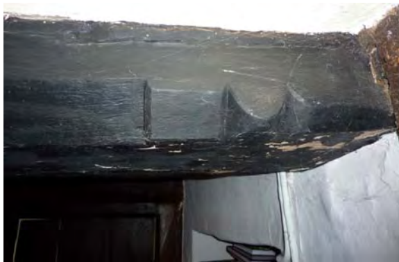
Detail of carved stops on beams; detail of bedroom door [01-01] and jamb
