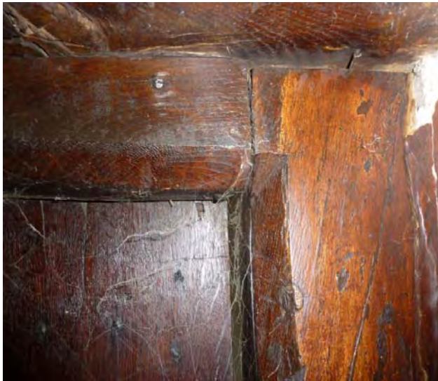
Detail of carved stops on beams; detail of bedroom door [01-01] and jamb
