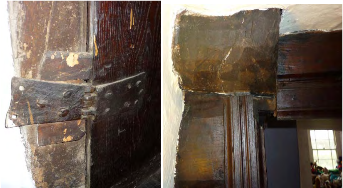
Detail of butterfly hinge on attic stairs door; cut off beam and later doorway made to fit
