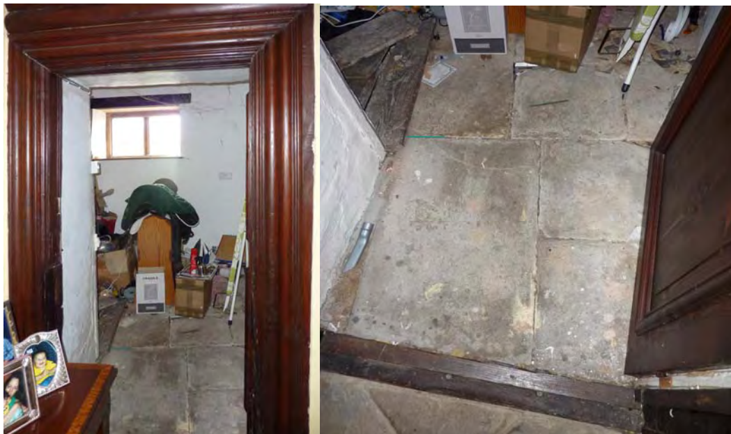
Lean-to looking north through bolection moulded doorway; flagged floor at an angle
