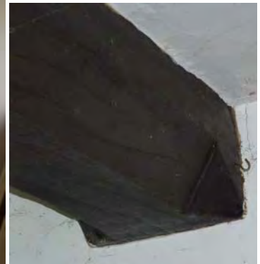
Looking south; detail of wide chamfered beam and rolled stop
