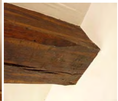
Kitchen looking onto passage; chamfered stop 18 th century
