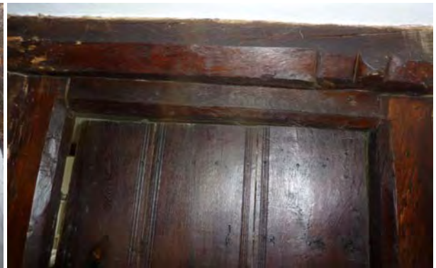
Detail of carved stops on beams; detail of bedroom door [01-01] and jamb
