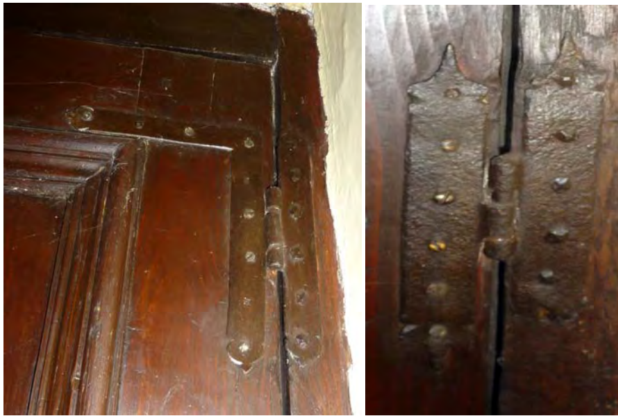
Cupboard under staircase & hinge; Sitting Room door and hinges
