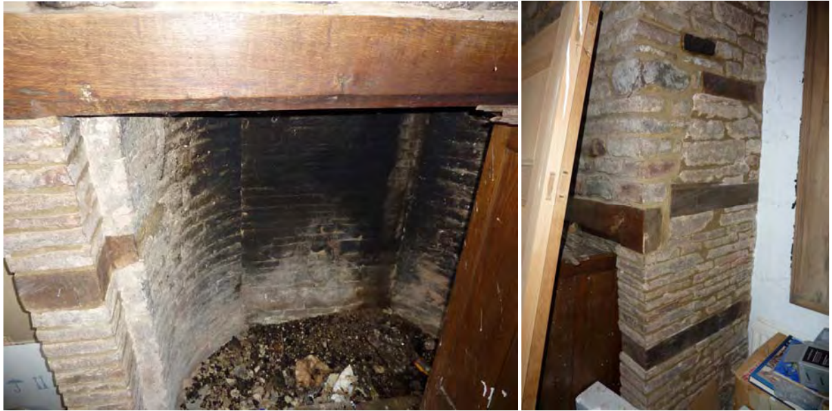
Rebuilt fireplace; 18 th century cupboard with modern shelves; doorcase with modern copied door, timber and sloping wall infill
