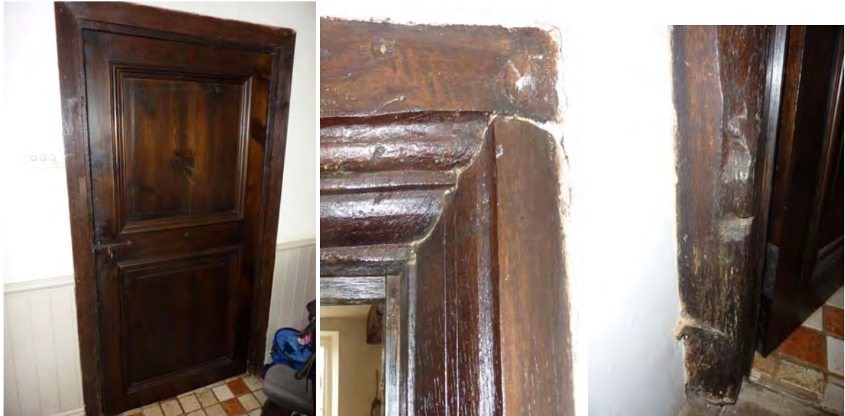
Kitchen door (modern copy) and detail of doorcase; carved stop on door jamb
