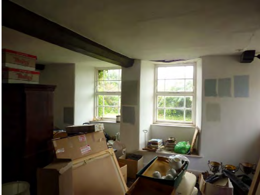
Looking south; detail of wide chamfered beam and rolled stop
