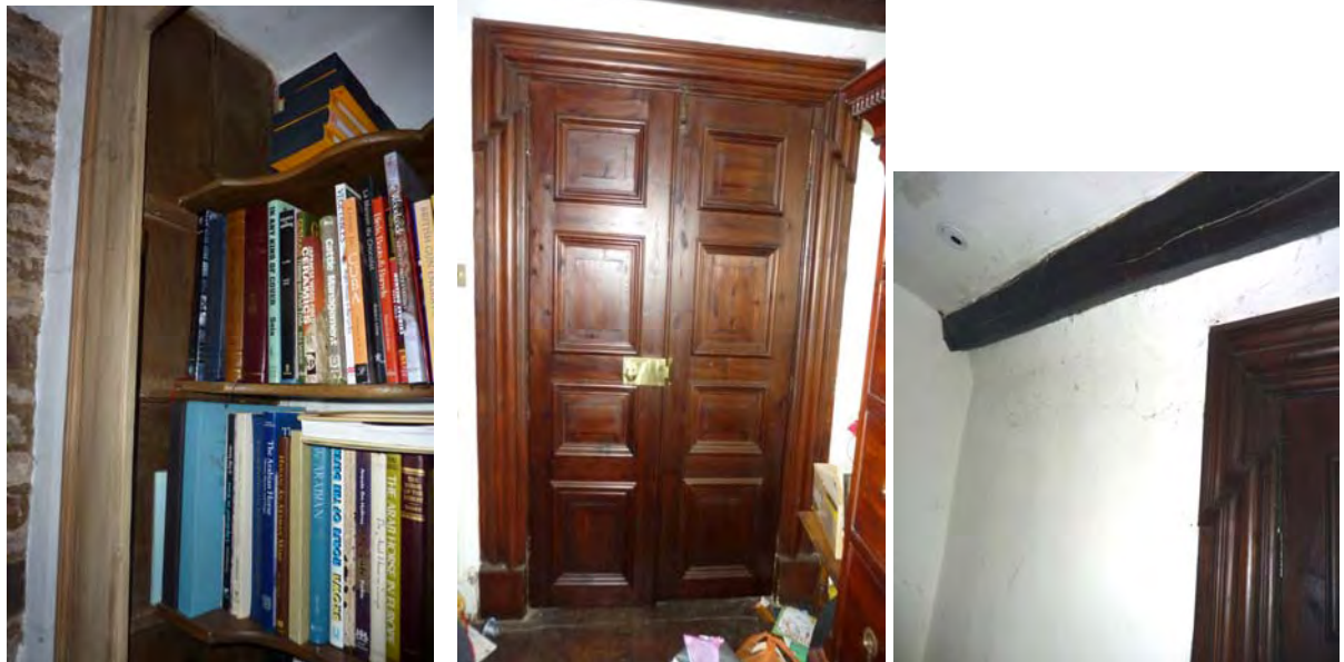
Rebuilt fireplace; 18 th century cupboard with modern shelves; doorcase with modern copied door, timber and sloping wall infill
