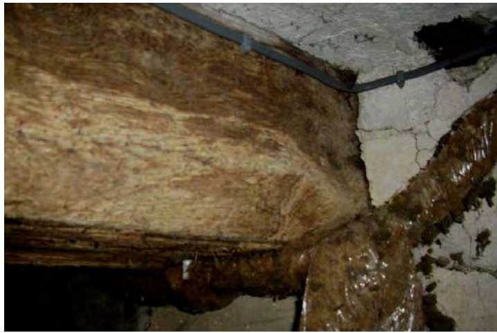
Chamfered beam and stop, similar to that in parlour above; cellar stairs (B Jones)
