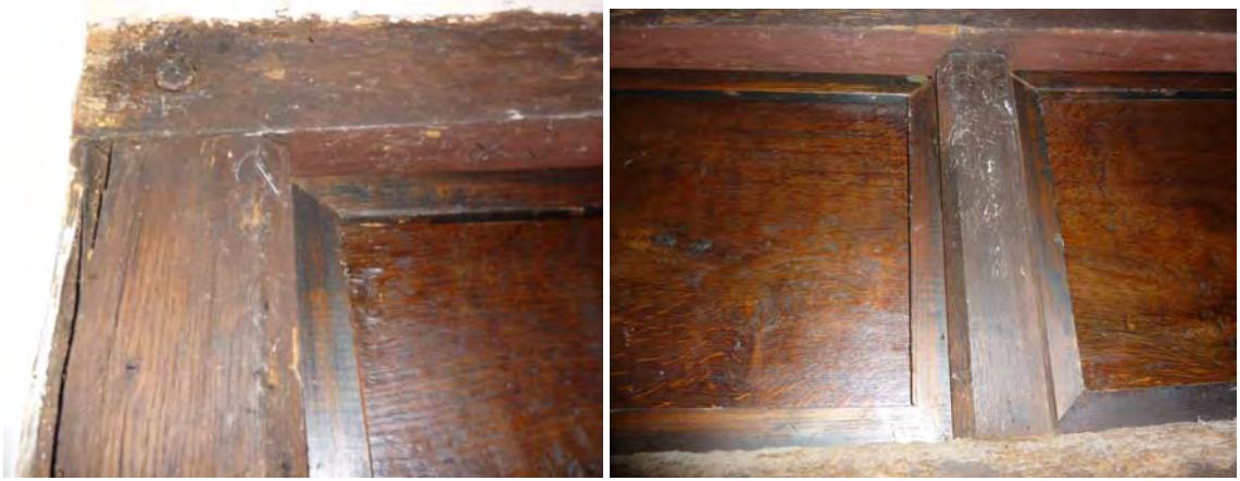
Detail of panelling above eastern doorway; weathered jamb; Hall door (modern copy) and door jamb
