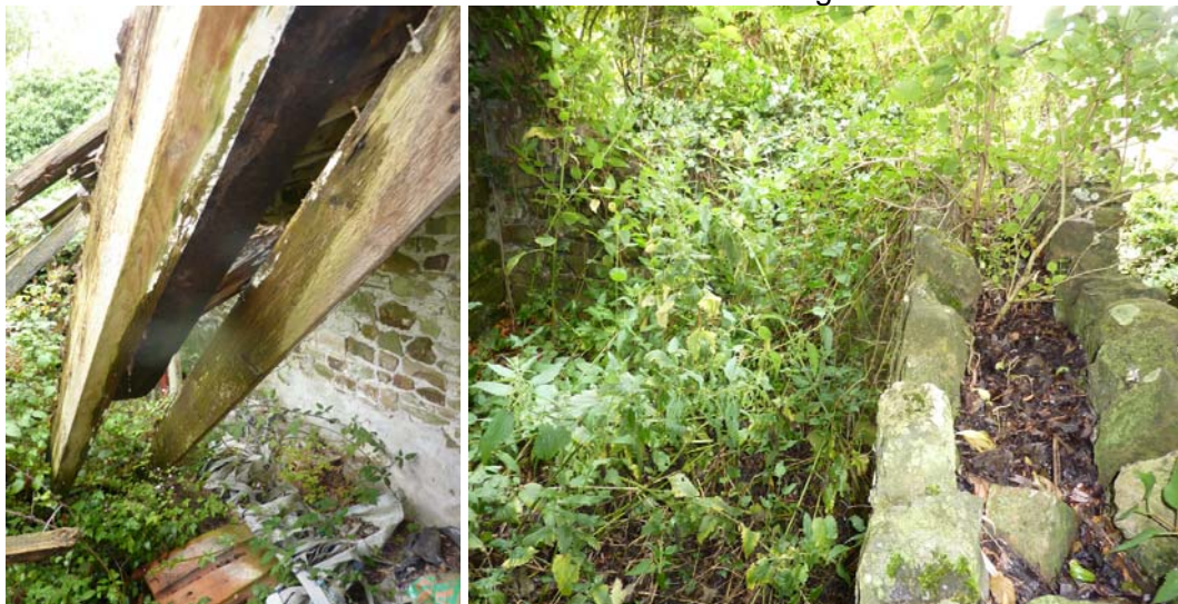
Garage north front; interior with collapsed roof truss & stone trough and former structure to south of the 2 buildings
