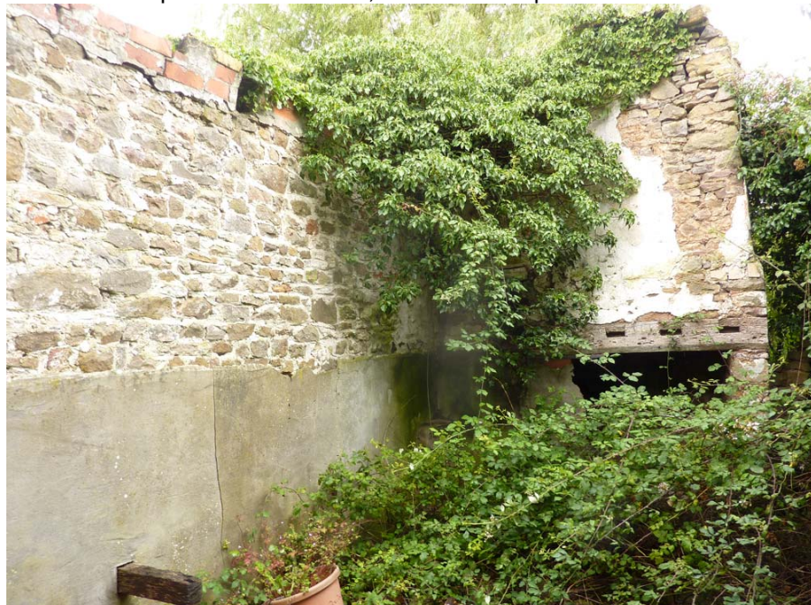
Interior rendered up to door level level; remains of fireplace with re-used timber lintel
