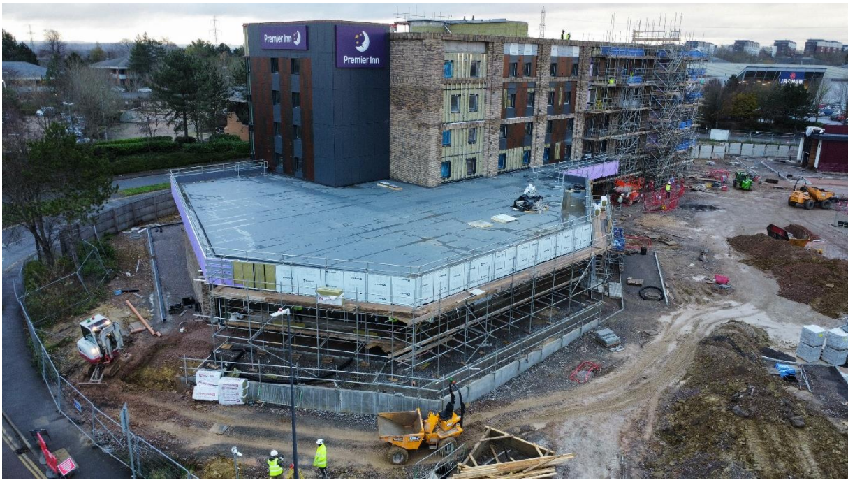
Image 6 – Photo of Fox Den Road scheme under construction (P20/05916/F)
